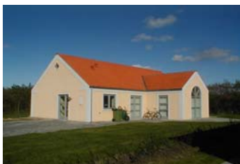
Figure 3. Danish low energy single-family house situated in Lemvig. The gross floor area is 145 m 2 (net area is 115 m 2 ). The area of windows and doors is 26 m 2
