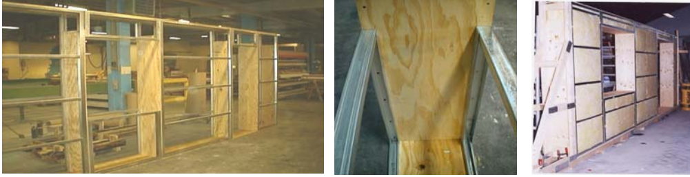
Figure 1. Typical light-weight exterior wall element with a load-bearing plywood and steel frame. Notice that there is no steel going through the wall element, and the studs is only placed around openings. Thereby the thermal bridge effect is minimal.
